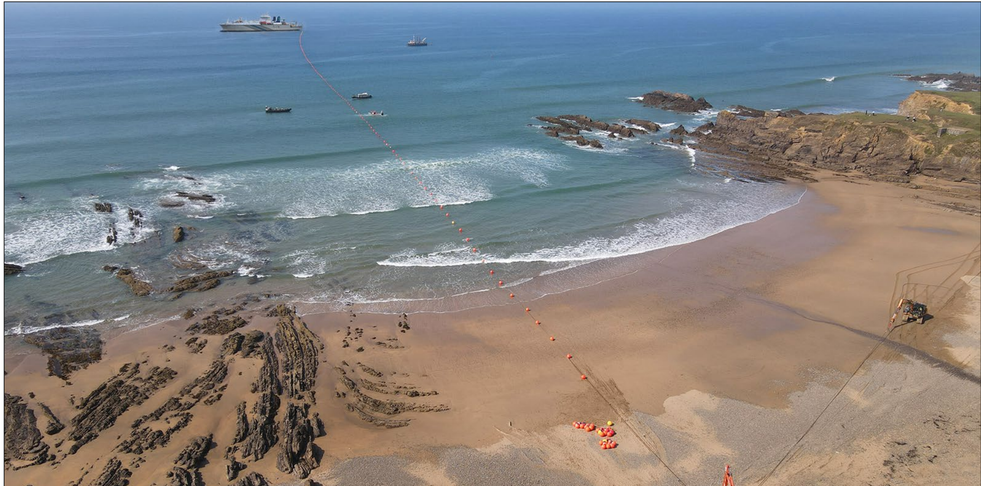
During a traditional cable landing, SubCom Reliance Class ships pay out cable as machines and operators pull from shore. Guard vessels stand by.
