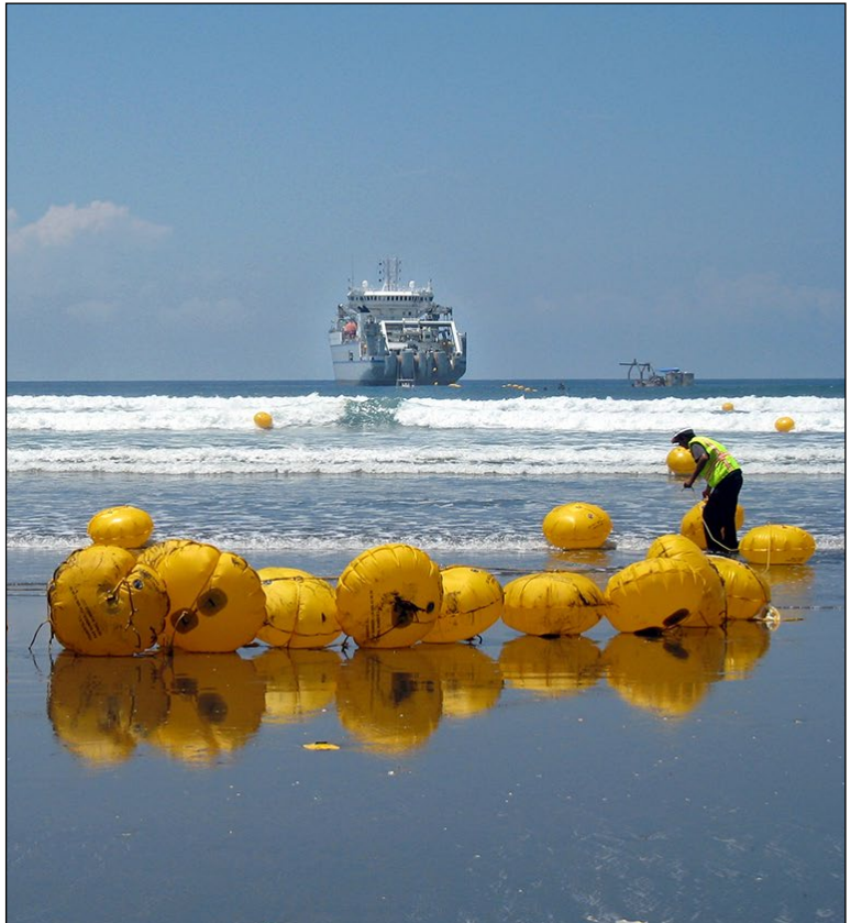
Collecting cable floats during a beach landing.
